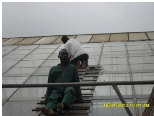
Fig 1. Manual Cleaning Procedure at the International Institute of Tropical Agriculture (IITA), Ibadan, Nigeria.
