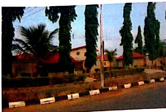
Plate 1.1: Wall Fence around Private Residence H
