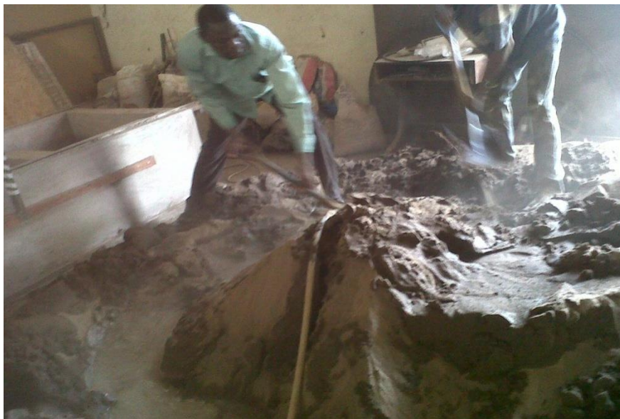
APPENDIX XIV: Picture of Soil Mixing Operation
