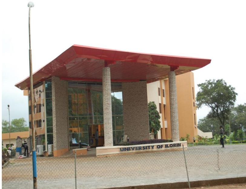
Plate 17: Entrance to Senate Building
