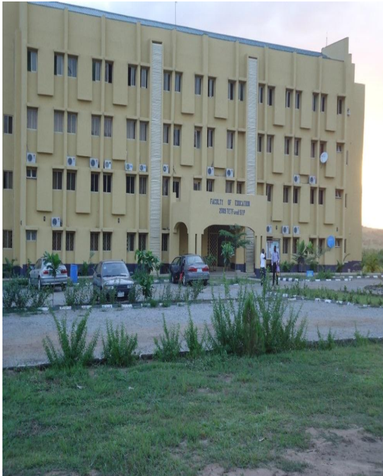
Plate 11: Faculty of Education 4-Storey Complex
