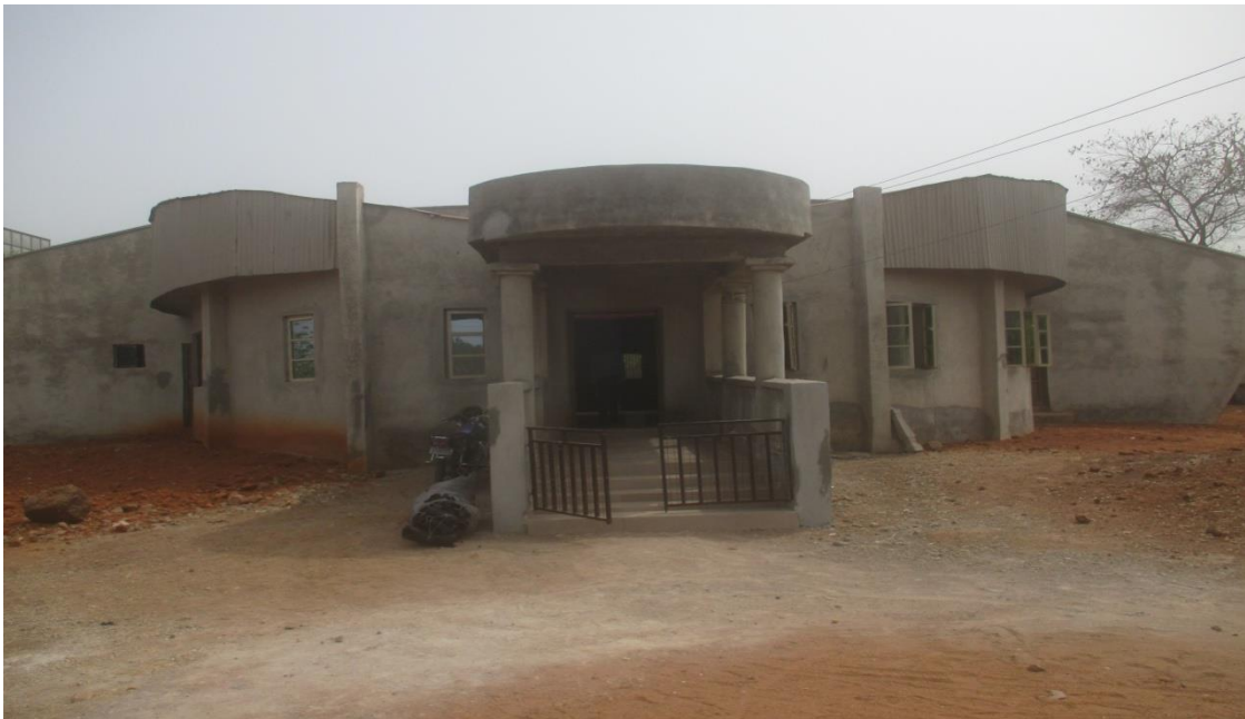
ECWA Ìgbàjà DCC Secretariat (under construction) Source: Picture taken by the Researcher at Igbaja on 28/06/2016
