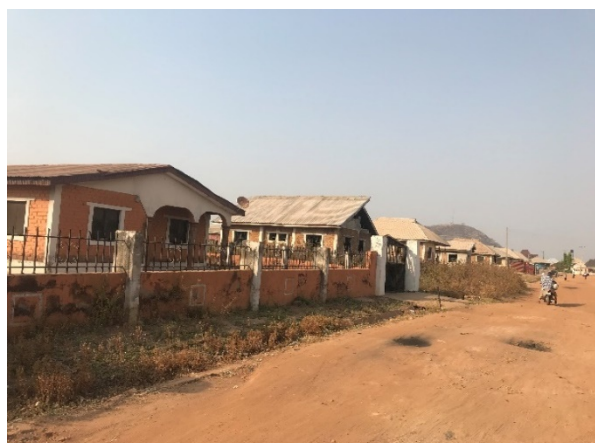
Plate 2: Road and drainage condition in harmony housing estate Source: Author's Field Survey, (2021)
