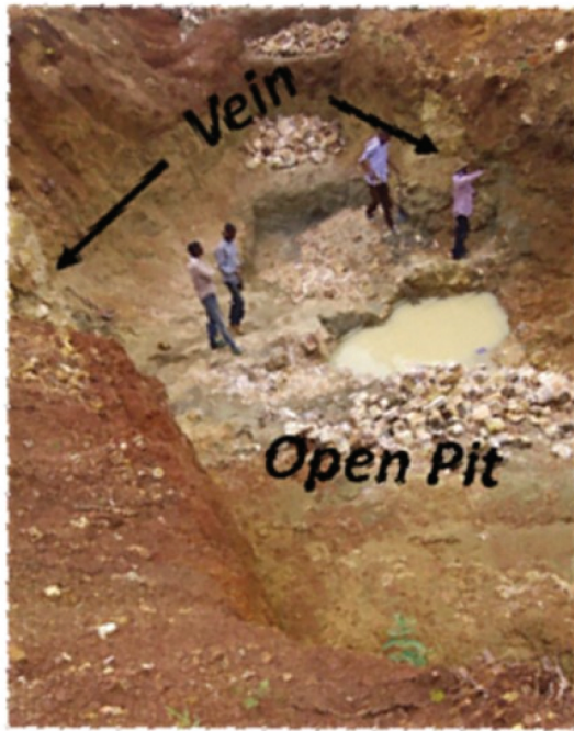
Figure 4. The image of a pit dug to confirm the presence tantalite-mineralised vein detected by resistivity survey.
