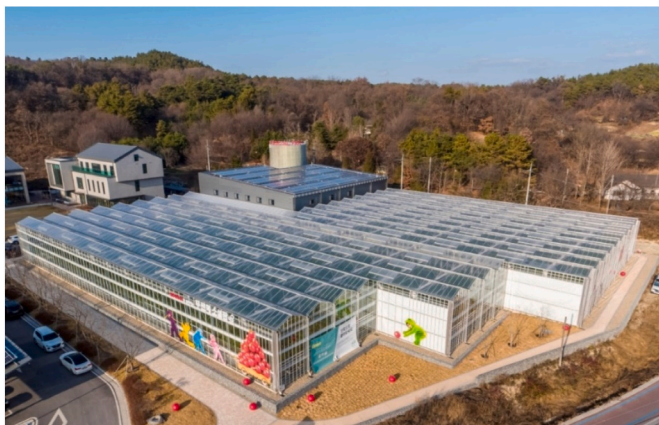
Fig. 4. Aerial view of the Yeoju experimental greenhouse.
