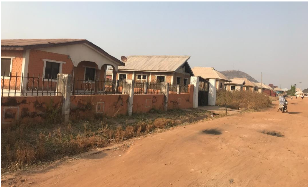
Plate 16.2: Blocked drainage and bad road in Harmony Mass Housing Schemes Ilorin
