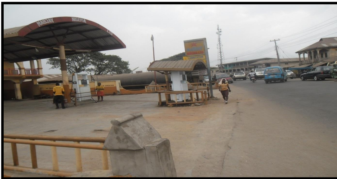
Plate 4: Petrol filling station without setback to road
