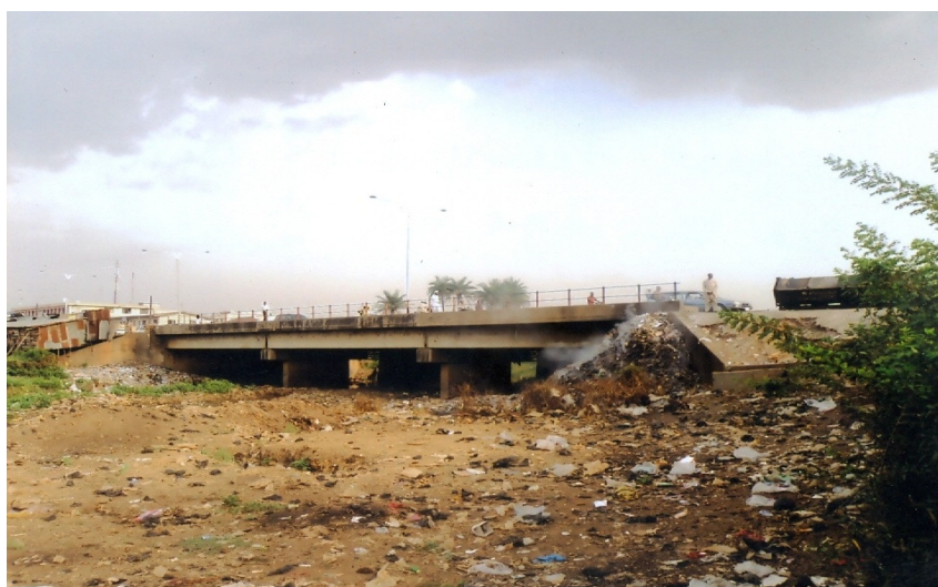
Plate 2: Refuse dumpsite, under the Bridge at Railway station, Ilorin
